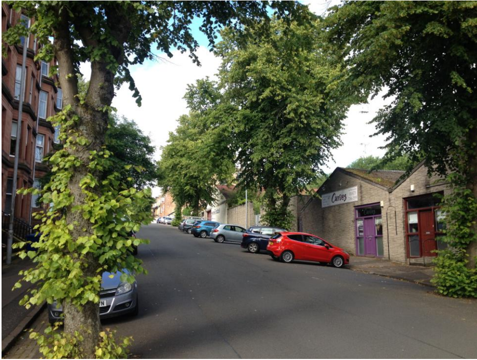
Photograph 5 : Robertson St : Business premises in near proximity to Residential tenement block.
